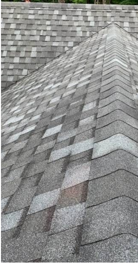
Roof-covering material — inspection view
