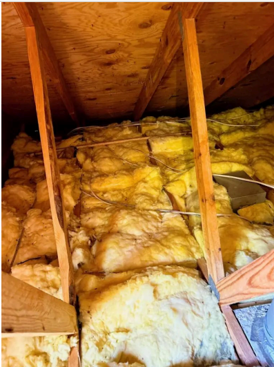
Insulation type observed — inspection view
